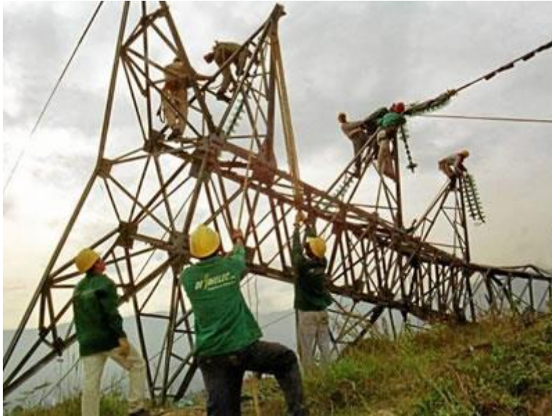
Figure 7. Civil workers repairing a tumbled electric tower in Tumaco (Colombia).
